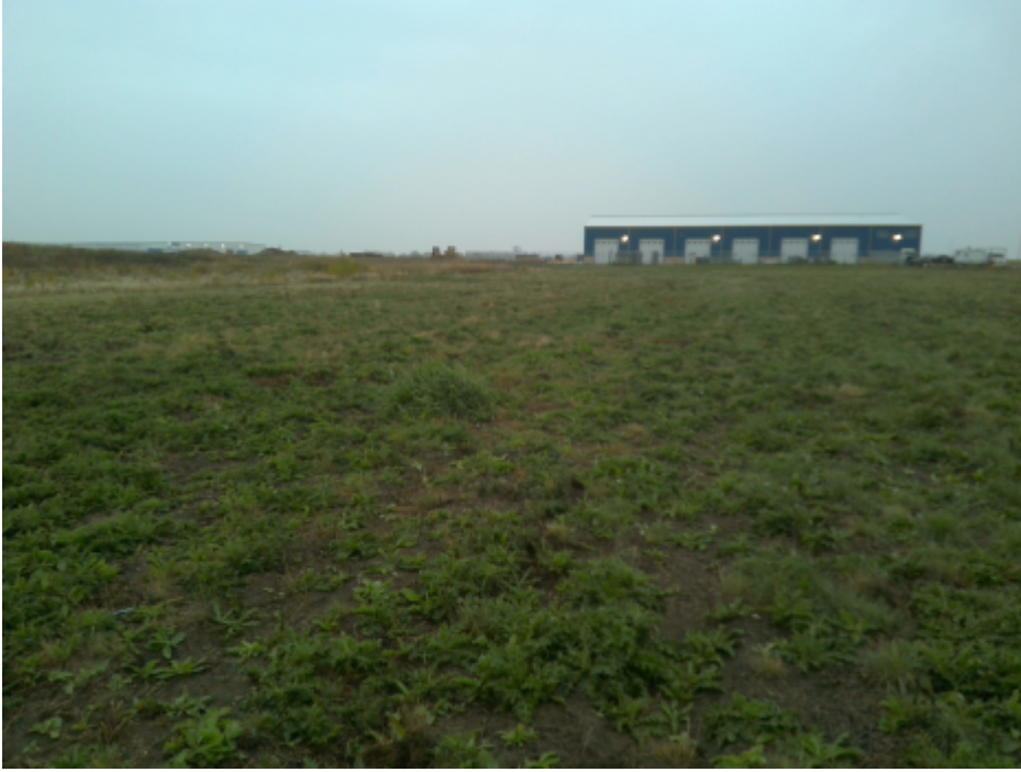
Photo 1 wcab009_u facing southwest
