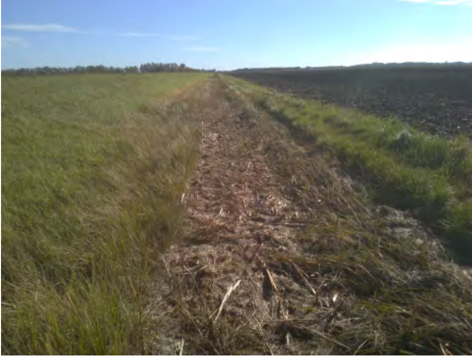
Photo 1 Photo facing east
