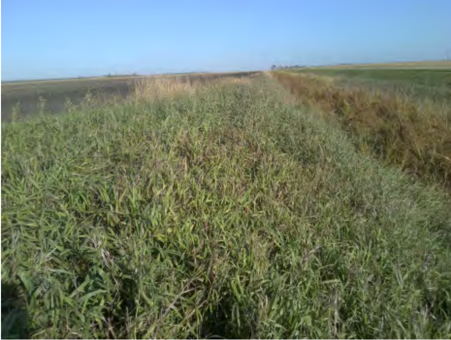
Photo 1 Photo facing north
