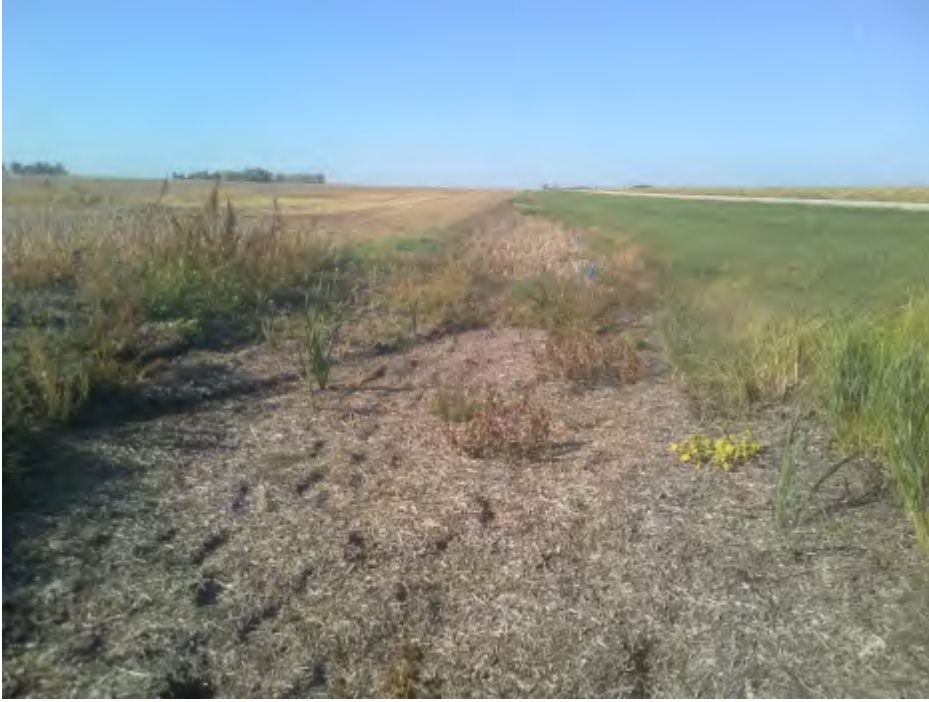
Photo 1 wcab005e_w facing west
