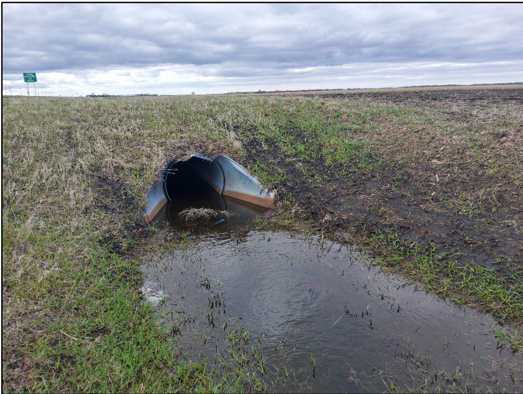
srig001e Downstream Facing South
