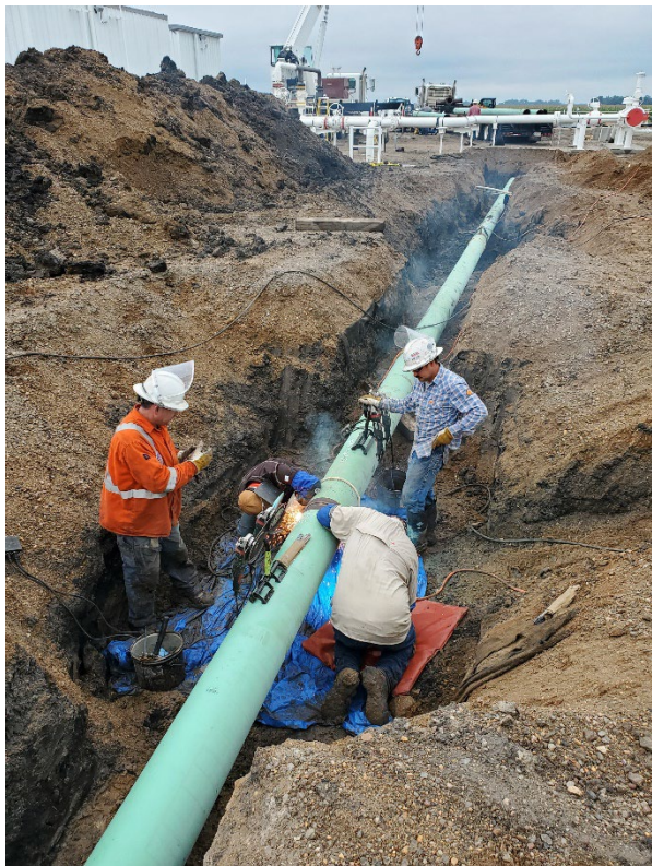
Date: 8/29/2024 Location: Mapleton Compressor Station. Notes: Welding underground piping.
