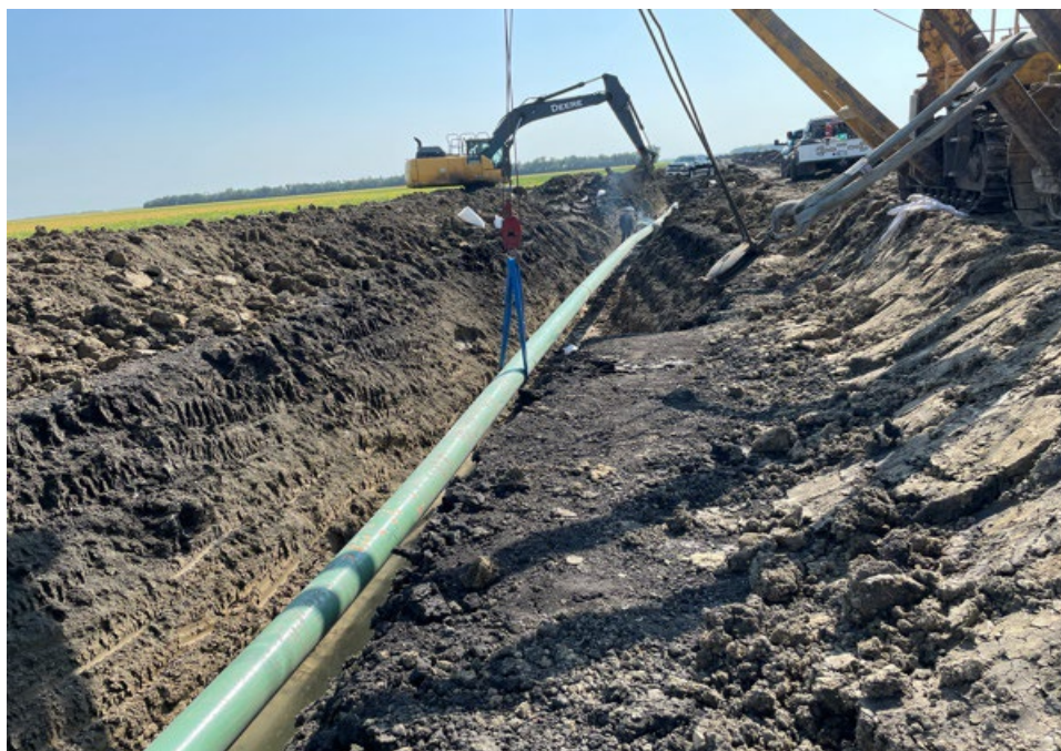
Date: 9/14/2024 Location: Sta. No. 1545+00 and Bore 37. Notes: Tie-in activities near Bore 37.
