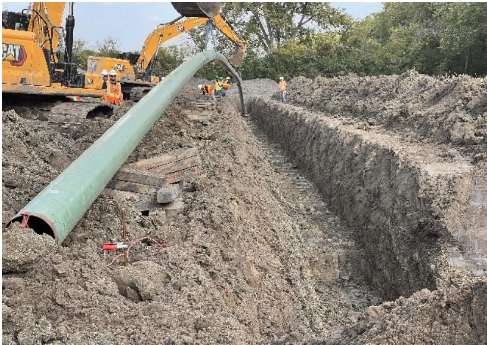
Date: 9/13/2024 Location: Sta. No. 1817+00 Notes: Lowering activities on the construction right-of-way.
