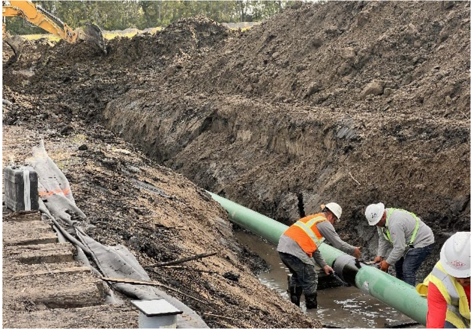
Date: 9/16/2024 Location: Sta. No. 1810+00 Notes: Coating activities at wetland wrib013 on the construction right-of-way.
