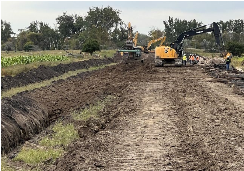
Date: 9/23/2024 Location: Sta. No. 1826+00 Notes: Backfilling activities on the construction right-of-way.
