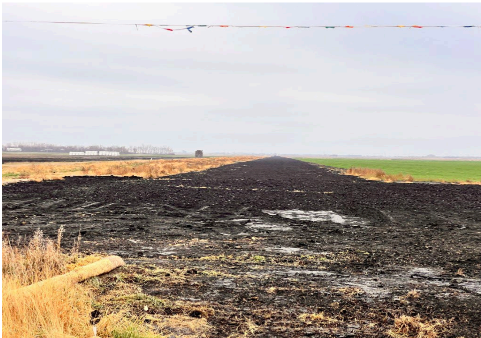
Date: 11/02/2024 Location: Sta. No. 2238 +00 Notes: Looking west across construction right-of-way.
