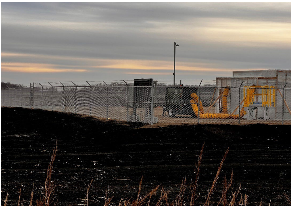
Date: 11/14/2024 Location: Valve Site 7 and MDU-Wahpeton Border Station. Notes: Completed security fence.
